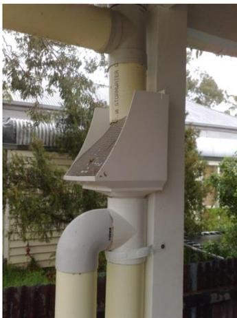
The water is collected from the front half of the roof, flows through a leaf eater and a first flush diverter, and then into the tanks.
